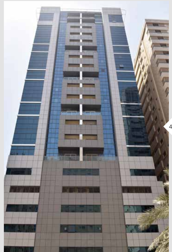
AL KHAN 6 Project: 21 Stories No. of Unit: 195 Residential Units Studio-1 BR, 2BR
