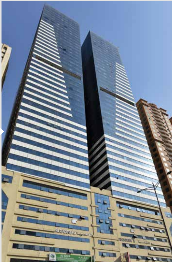
AL QADISIYA Complex 4 Towers Project: 25 Stories No. of Unit: 630*4=2520 Residential Units Studio, 1 BR From 650-780 Sq.Ft for A1. 650-780 Sq.Ft for A2
