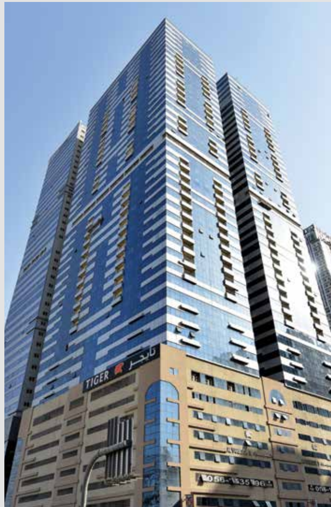
AL YARMOOK Complex 4 Towers Project: 45*4=180 Stories. No. of Unit: 630*4=2520 Residential Units Studio, 1 BR From 538-740 Sq.Ft for A1. 538-750 Sq.Ft for A2
